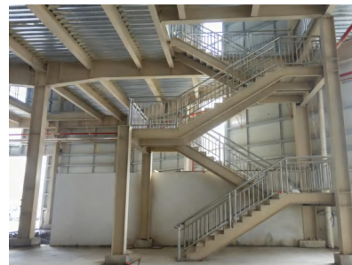
Meilin Construction Site's staircase
