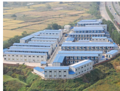
Dawang Construction Site
