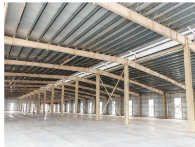
Meilin Construction Site's interior view
